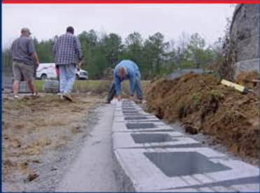
(5) Blocks are aligned as desired. If wall is straight, use a string line.
