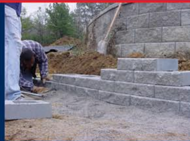
(7) Additional courses of Geostone blocks are placed on the base course in running bond. Be consistent in setting the batter (set back) in each course.
