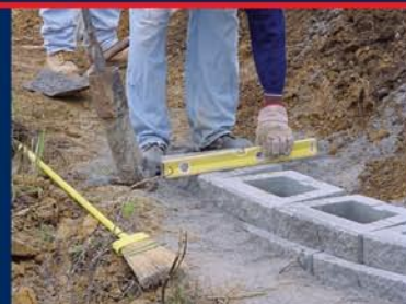
(11) Stepping Up is a method used to follow a slope up hill. The base course runs into the ground as shown while the course above continues on. Make sure to level each footing block in the step up procedure.
