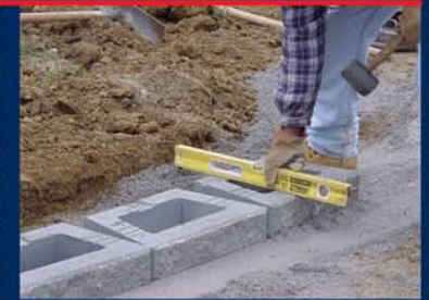
(8) When 2 to 4 courses of block have been placed in your wall and properly aligned you will overfill (slightly) the core of the blocks and two feet behind the wall with #67 crushed stone every 2 to 4 courses. Plate or hand compact the stone until level with the top of the block.
