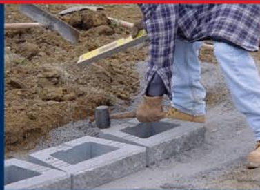
(6) Finish leveling. Using a 2 foot carpenter's and a rubber mallet, level each block front to back and side to side with the adjoining block.
