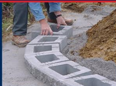
(10) Adding a curve can be achieved easily due to the shape of the block and it not being hindered by lips or pins.
