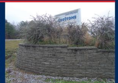
(12) Finish the wall with the Wall Cap product. Adhere Wall Cap to the last course of block with outdoor construction adhesive.
