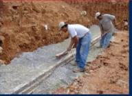
(11) Sweep <u>ALL</u> rock and gravel for the tops of the blocks before laying down next course of geogrids. Any variance in height caused by rocks between courses will cause unsightly gaps. Backfill area should encompass entire proposed grid length area.
