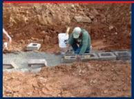
(5) When laying the first course, level the block front to back and side to side with a two foot carpenter's level. It is very important that the first course be level and placed on a compacted footing.
