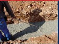
(2) The footing depth will vary based on the the height of the wall. Rule of thumb is 1 inch of embedded block per vertical foot of wall height is required. Place four to six inches of crushed rock (#78 or #8910) in the footing and level for the wall foundation.
