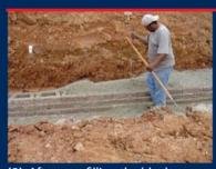
(9) After core filling the block, use a rod to drive down into the cores to assure a thorough core fill. Backfill should be level to top course of block
