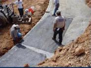
(12) Next lay out the georids. Their length will depend on the wall height. Rule of thumb is no less than 75% of wall height ( no shorter than 4") and no less frequent than every 2 vertical feet.
