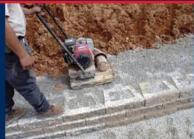
(10) Compacting the backfill is very important. This provides additional resistance to pressures exerted on the wall and prevents settlement. Repeat this process after each backfill.
