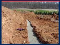
(1) Begin by digging a two foot wide trench. Excavate all loose soils and native rock until hard original ground is reached. The footing will be supporting the entire weight of the wall.
