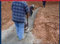
(3) As preparation of the footing continues, remove all large rocks and use a vibrating plate tamp to achieve proper compaction. Get footing as smooth level, and compacted as possible.
