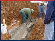
(4) Run a string line for straight walls. This willlleip in the align ment of the first course. Use a cement trowel to smooth out base prior to setting the first block.
