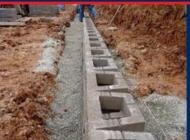
(7) Align and batter each course prior (8) It is recommended that the cores to core filling with rock. Batter means setting each course back 1/4 - 1/2 inch behind the course below as seen in the picture above. On straight walls, use as a string line. In curves, visually align the wall to achieve the desired appearance.
