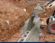
of the block be filled with a #67 or #78 stone no less frequently than every three courses. This same stone is recommended for the backfill as
