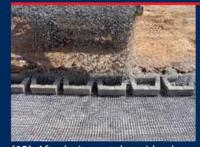
(13) After laying out the grids, place another course of block down on top of the grids, align, then core fill and backfill. It is important that the grids be stretched tight prior to placing rock fill.
