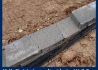
(14) Finish the wall with the Wall Cap product. Adhere Wall Cap to the last course of block with outdoor construction adhesive.
